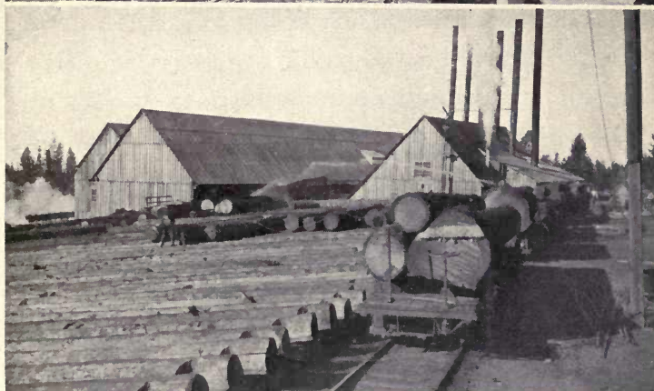
Figure 64. Logging in California. Powerful steam engines pull the logs from the woods to the railroad and load them on flat cars. Photo by the author.
